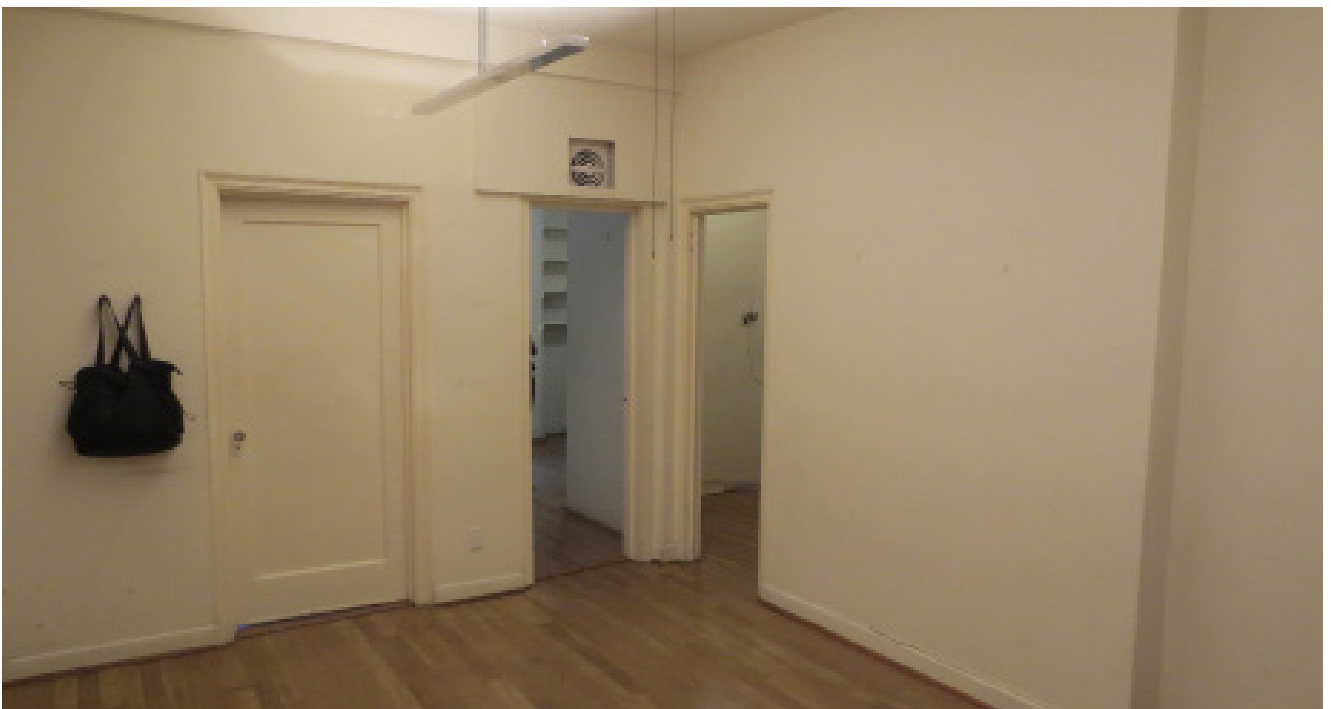
Without access to natural light, the original space was too dark. Photo courtesy of PJCArchitecture.
