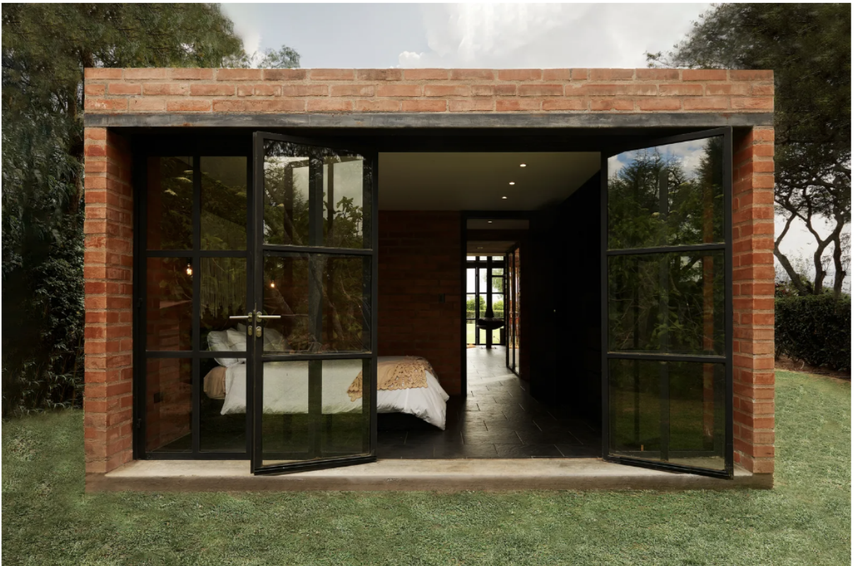
Air conditioning and heating systems are not typically used for residential spaces in Ecuador, according to Nandar. “The brick is a thermal mass material that absorbs heat from the sun throughout the day,” she explains. “And the glass bridge, when in an open position, creates a cross air ventilation that helps to cool the two volumes during the hot days.” Juank Paredes Photography
