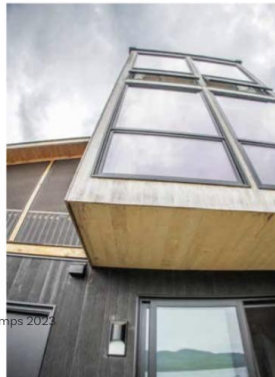
Below: Japanese-charred wood, on the home’s exterior, weathers well and is pest resistant.
